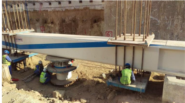
Fig. 11. Pile load test set up with two reaction piles
