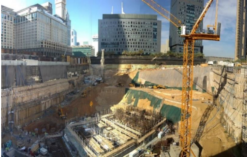
Fig. 12. The new tower under construction
