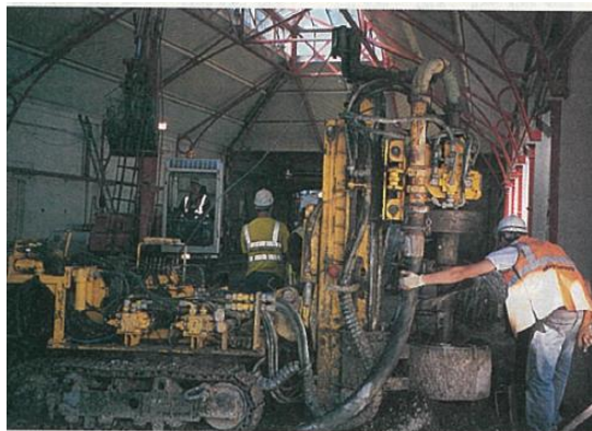
Fig. 4. CFA rig in low headroom mode
