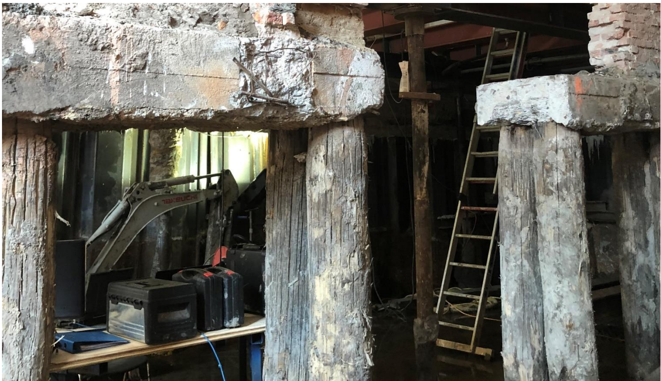
Figure 4: Inspection of an Existing Timber Pile Foundation
