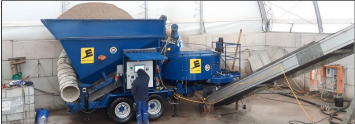
Fig. 2: Mobile mixing plant with a conveyor belt
