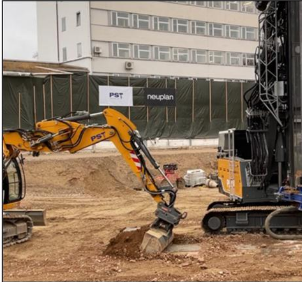
Fig. 6: Removing the drilled material
