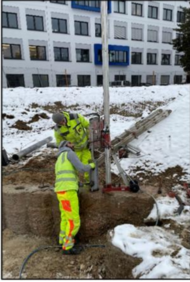
Fig. 11: Core Drilling
