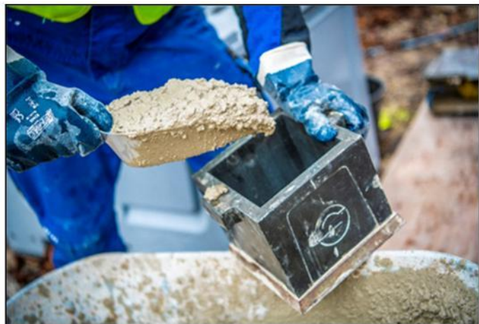
Fig. 9: Production of concrete cubes
