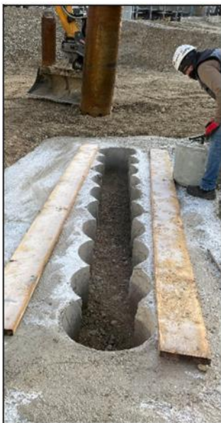
Fig. 3: Drilling template
