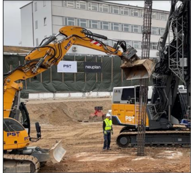
Fig. 7: Installing the reinforcement cage
