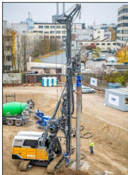
Fig. 4: Positioning at the drilling point and starting drilling process
