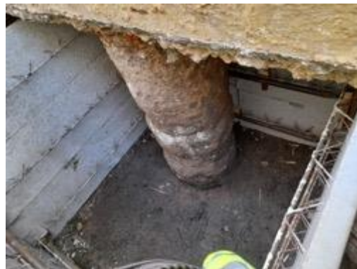
Fig. 1. Braced excavation around existing pile – Franki pile
