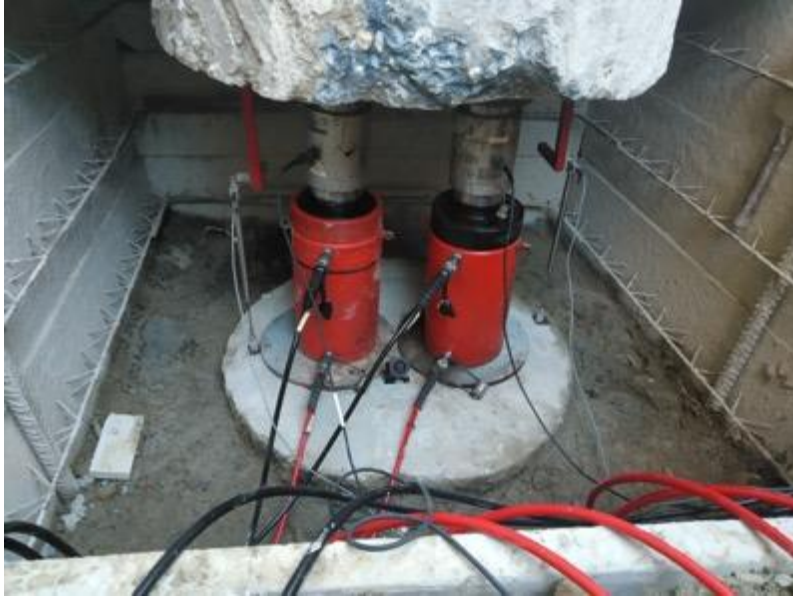
Fig. 4. Set-up for pile testing of working pile
