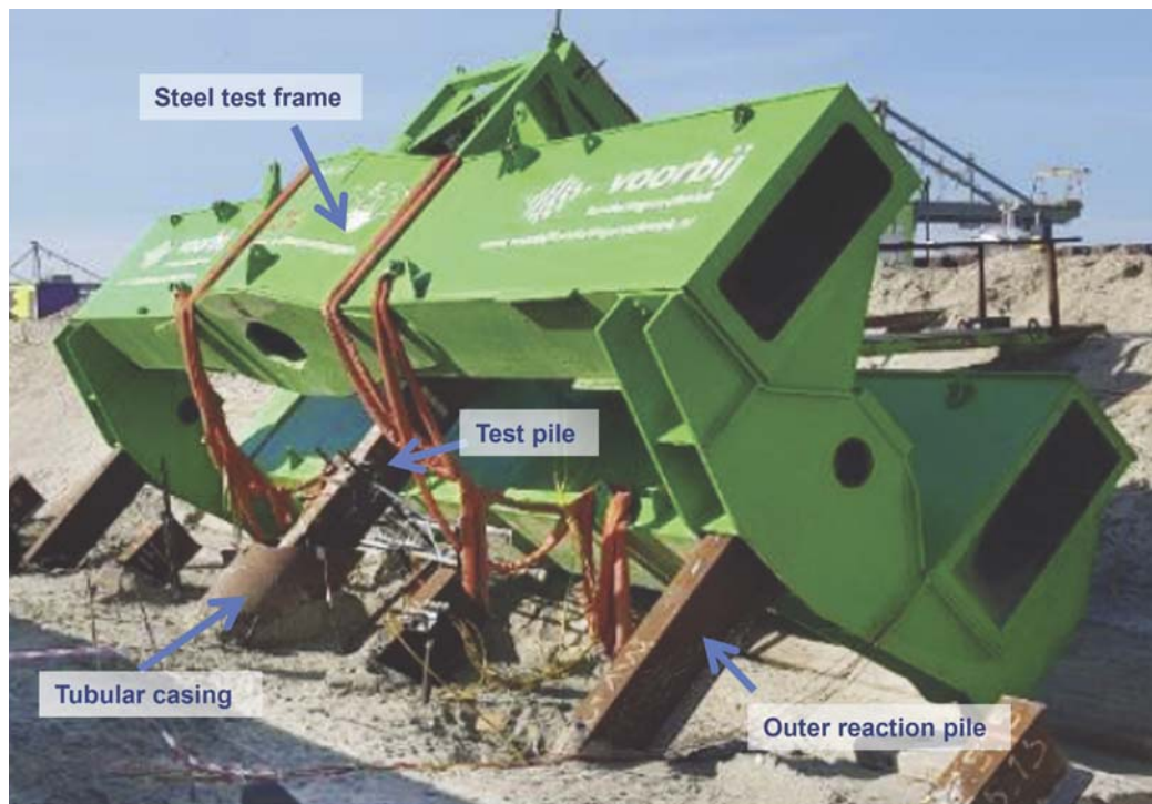
Figure 4 – Overview of test setup pile load test Mississippihaven.
