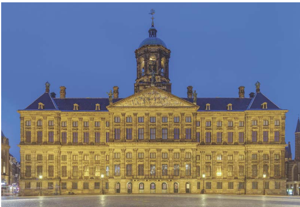
Figure 1 – The Royal Palace on Dam Square in the heart of Amsterdam was originally built on 13,659 timber piles. Over time, its foundation underwent significant restoration to address uneven settlements. During an extensive renovation in 1945, additional piles were installed to stabilize the structure. As a result, the palace now stands on a total of 13,681 piles, effectively extending its technical lifetime.
